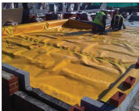
Figure A4.18 Gas membrane installed as part of foundation barrier (courtesy Industrial Textiles & Plastics Ltd)
