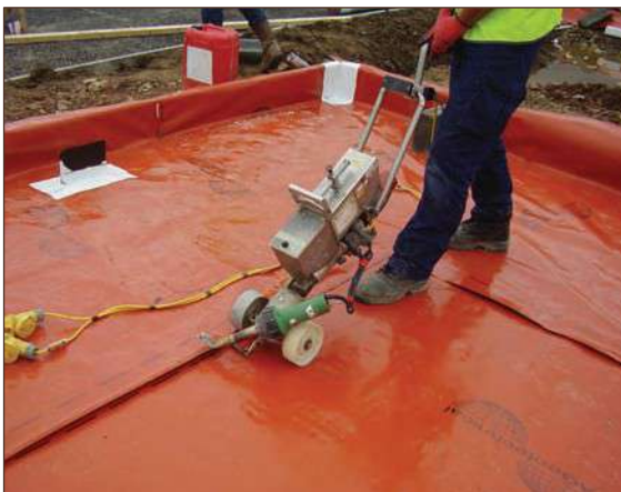
Figure A4.31 Extrusion welding (courtesy PAGeotechnical Ltd)
