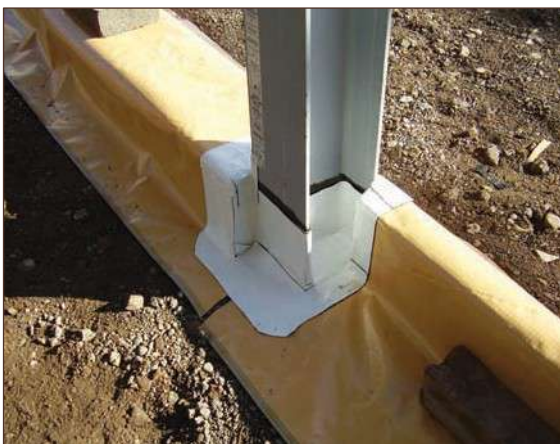
Figure A4.23 Complex column seal (courtesy PAGeotechnical Ltd)
