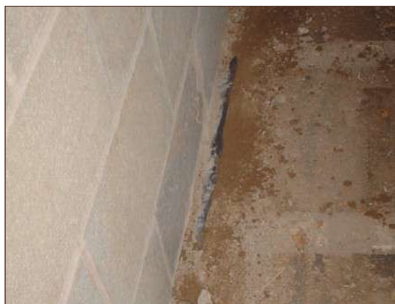
Figure A4.64 Insufficient length of gas membrane protruding through wall to overlap with gas membrane within building (courtesy Card Geotechnics Limited)
