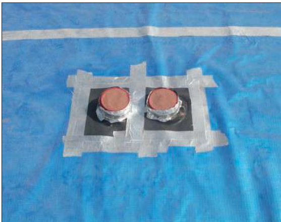
Figure A4.27 Top hats placed around service entries secured with jubilee clip seals. Top hats secured to gas membrane with double sided butyl tape (courtesy Hydrock)
